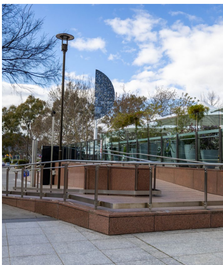
Accessible ramp to the Science Court and general public entrance.
