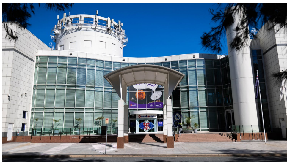
School group entry via the Ceremonial Entrance. An accessible ramp can be found on the left-hand side.
